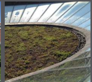
Harvard Business School Class of 1959 Chapel Boston, MA Extensive Green Roof
