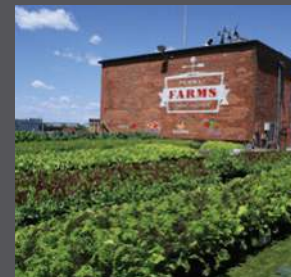
Fenway Farms Boston, MA Rooftop Farm
