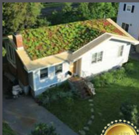
Private Residence Winchester, MA Extensive Green Roof
