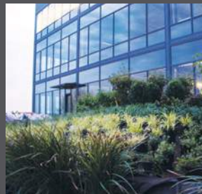
450 Artisan Way Assembly Row Somerville, MA Mixed-Use Roof Terrace
