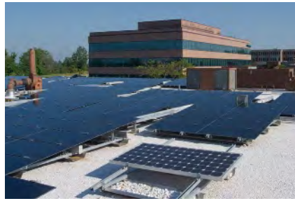
Rock-IT* All-White Reflective Roofing System Beneath Photovoltaic Roofing System
