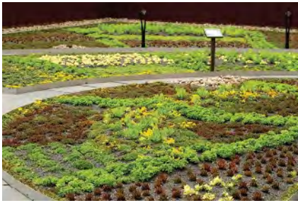
Extensive Vegetated Roofing System (Front)
