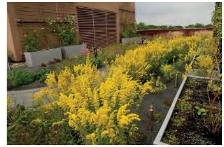
Extensive Vegetated Roofing System (Back)
