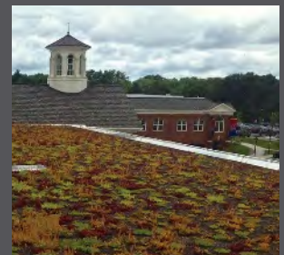
Natick High School Natick, MA Extensive Green Roof
