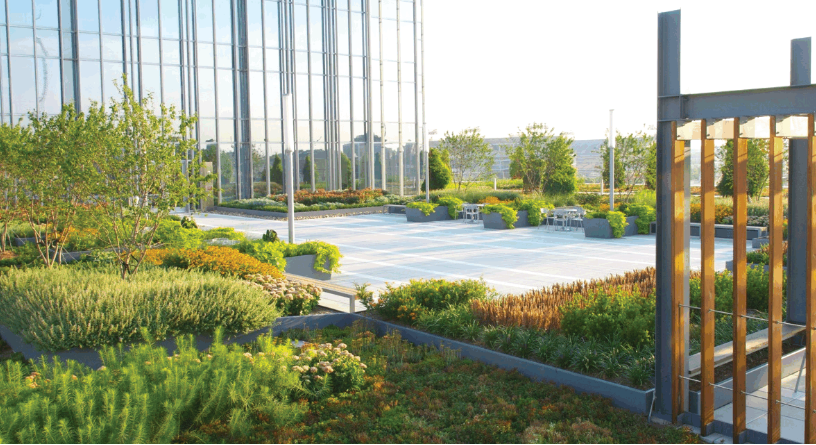
OPPOSITE: MUSIC CITY CENTER GREEN ROOF IN NASHVILLE
