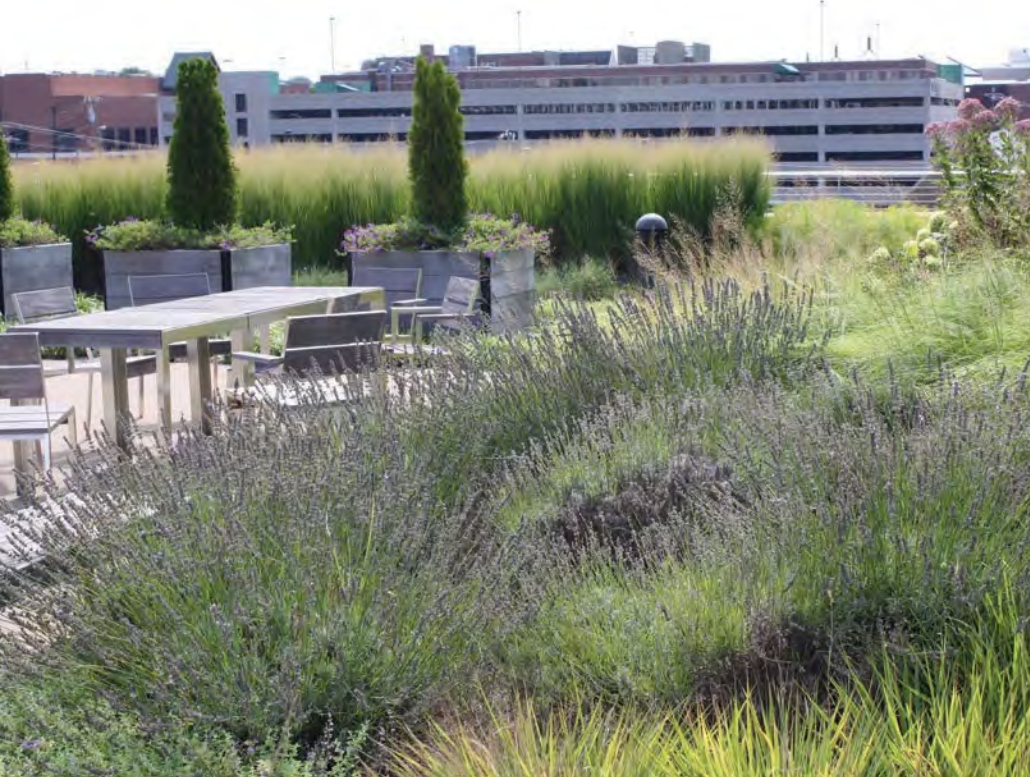
LEFT: CALIFORNIA ACADEMY OF SCIENCES GREEN ROOF IN SAN FRANCISCO, CALIFORNIA
