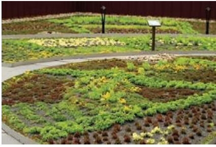
Extensive Vegetated Roofing System (Front)
